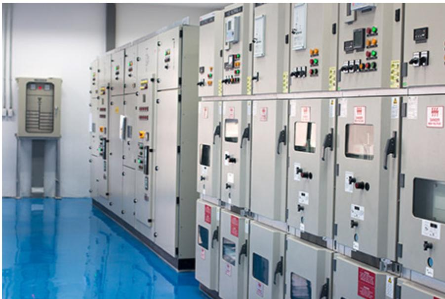
**Figure 1. Control Panel with Protection, Control and Monitoring Equipment**
