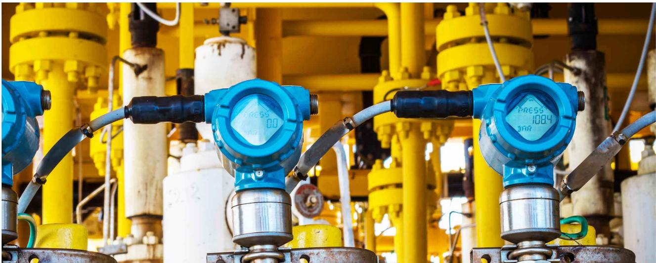
**Figure 1. Pressure Transmitters**
