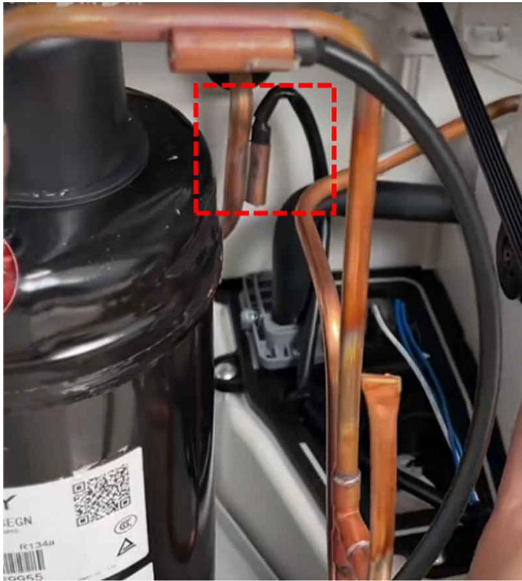
**Figure 1-5. Compressor Discharge Temperature Sensor Installation**
