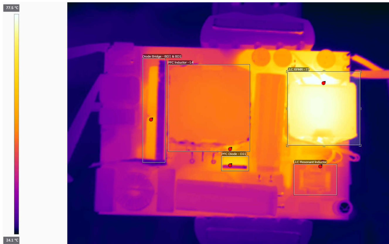
Figure 2-6. 230Vac, Full Load, Top Side Thermal Image
