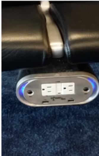
**Figure 1. Built-in USB Ports on Airport Terminal Seats**
