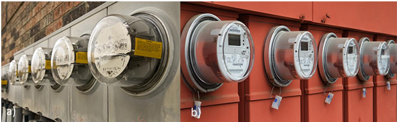
**Figure 1. Electromechanical Meters (a); and E-meters (b)**
