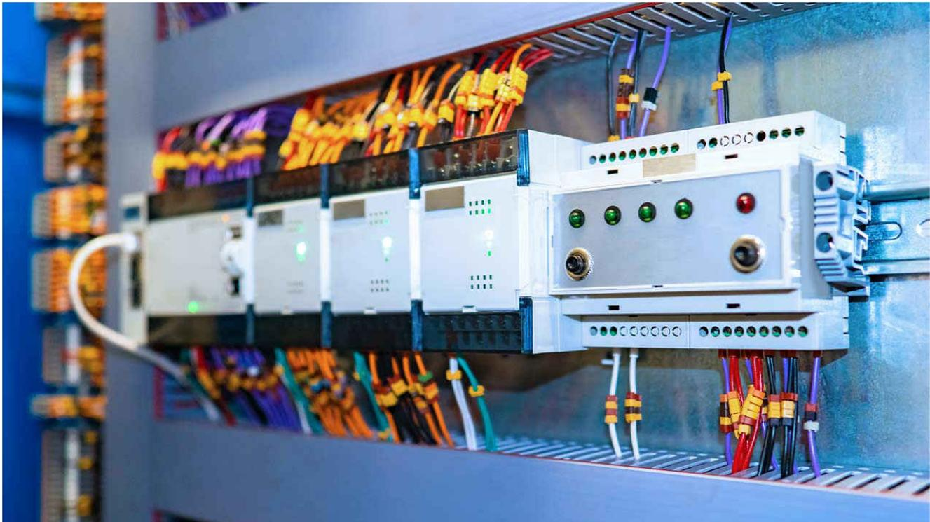
**Figure 1. A programmable logic controller in a factory environment**
